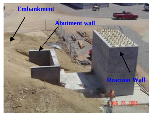
Fig. 5. Overall view of Abutment Wall During the Construction.
