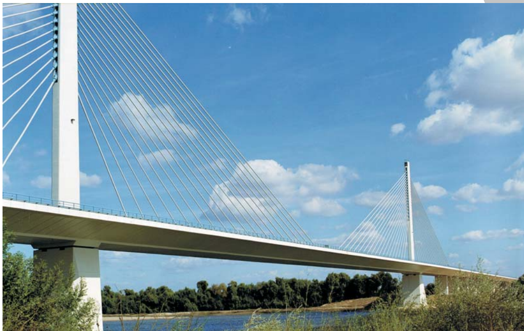
Ponte sul fiume Tago a Santarem isolato sismicamente con isolatori Algasism HDRB Bridge over Tagus river at Santarem (Portugal) seismic isolated with Algasism HDRB
